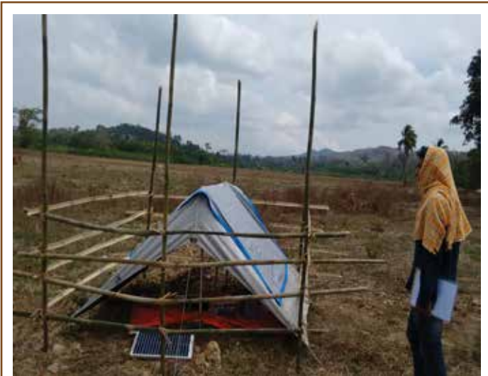
Figure 56 Installation of LMT unit at Ramnagar-I, Diglipur, North Andaman Islands.
